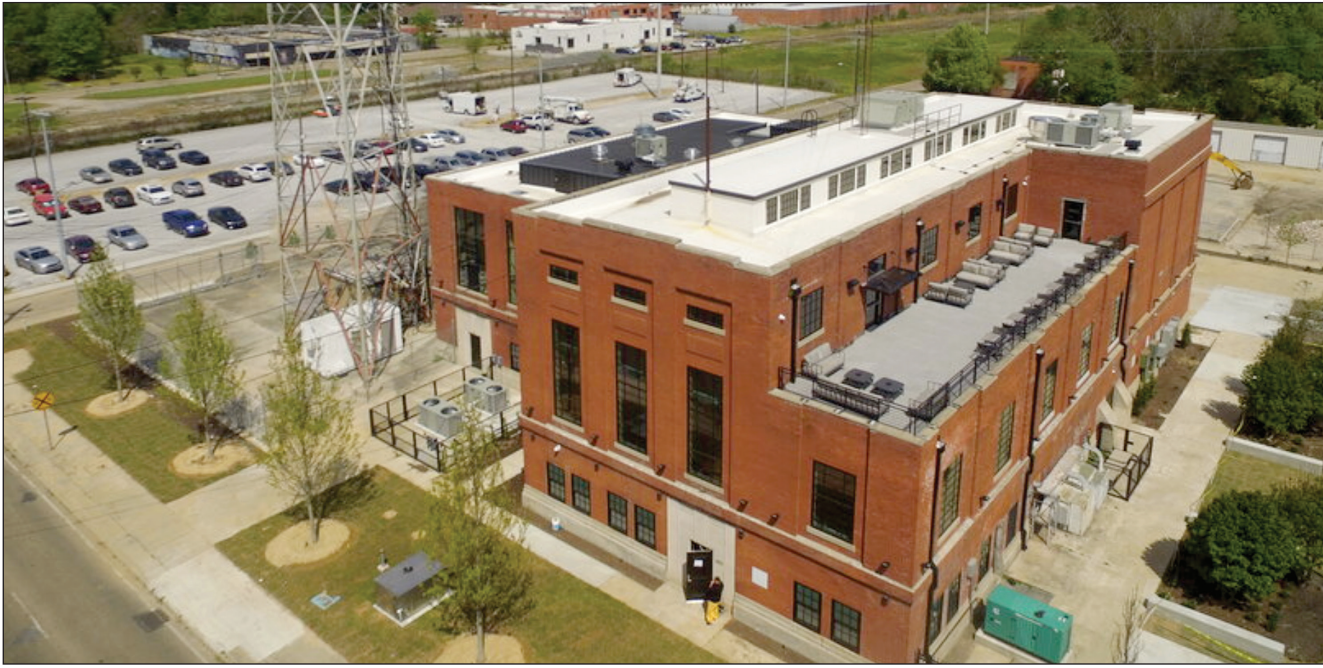
Electric Depot Phase II - 100 Multifamily Unite Project
