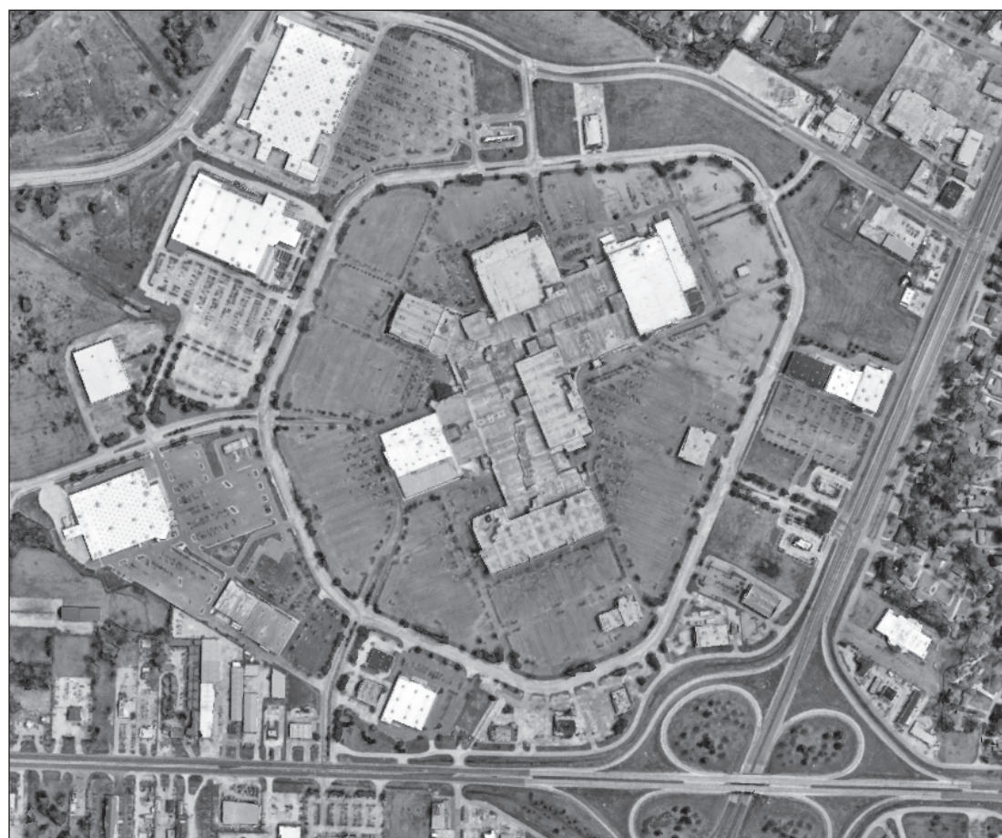
The old Cortana Mall will be the site of the new Amazon fulfillment center.
